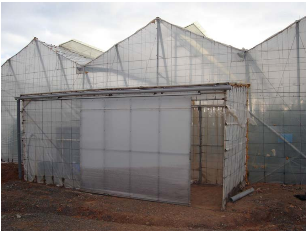
A screened greenhouse with double-door to prevent entry of Tuta absoluta . © A. Antón, IRTA, Spain.
